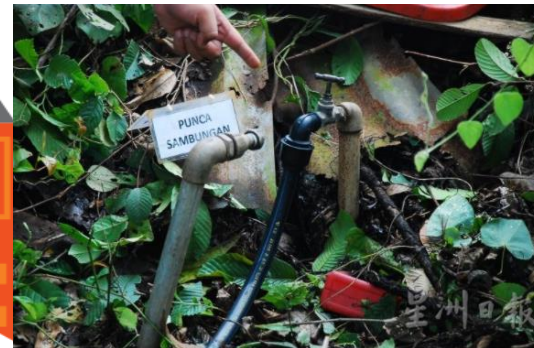
Someone used water pipes without permission to connect tap water for their own use without a water meter.
